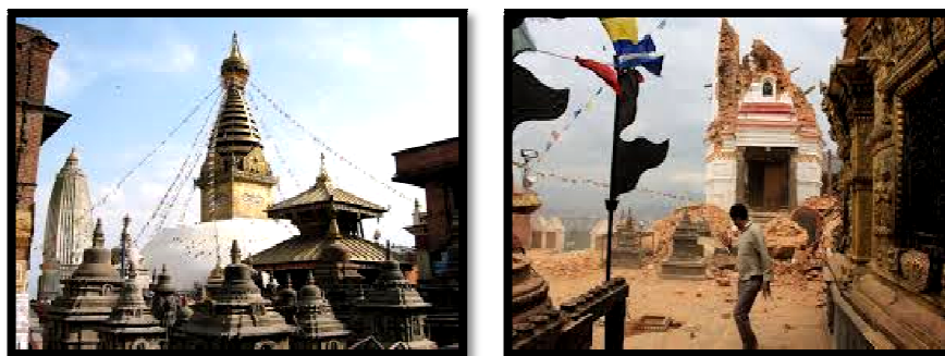
Figure 3: Condition of Swayambhunath Stupa Before and After Earthquake
