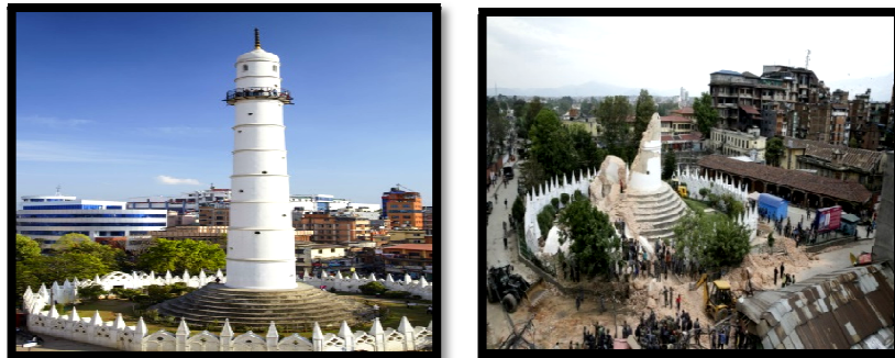
Figure 2: Condition of Bhimsen Tower Before and after Earthquake
